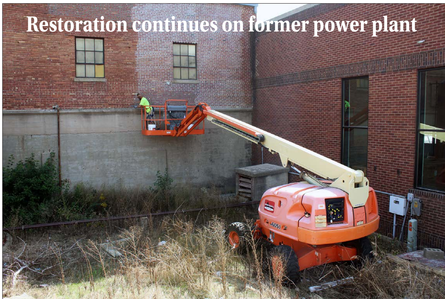
Mavis Fodness Photo/0908 Power Plant Work
