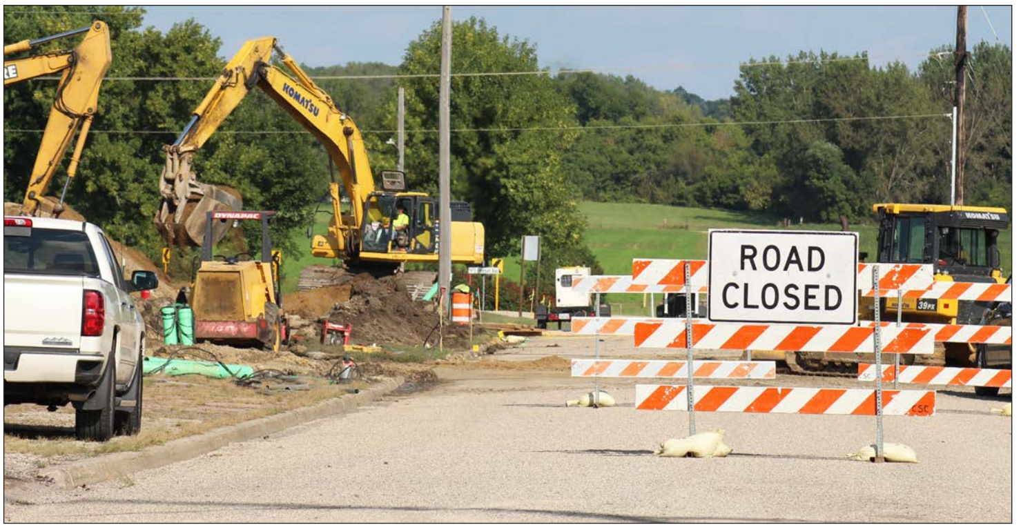
Mavis Fodness photo/0906 town square construction
