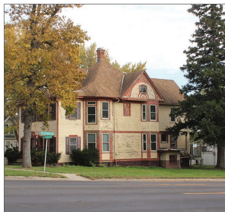
Lori Sorenson file photo/1023 condemned property
