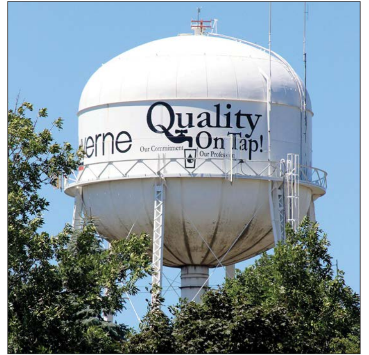
Lori Sorenson photo/0806 water tower
