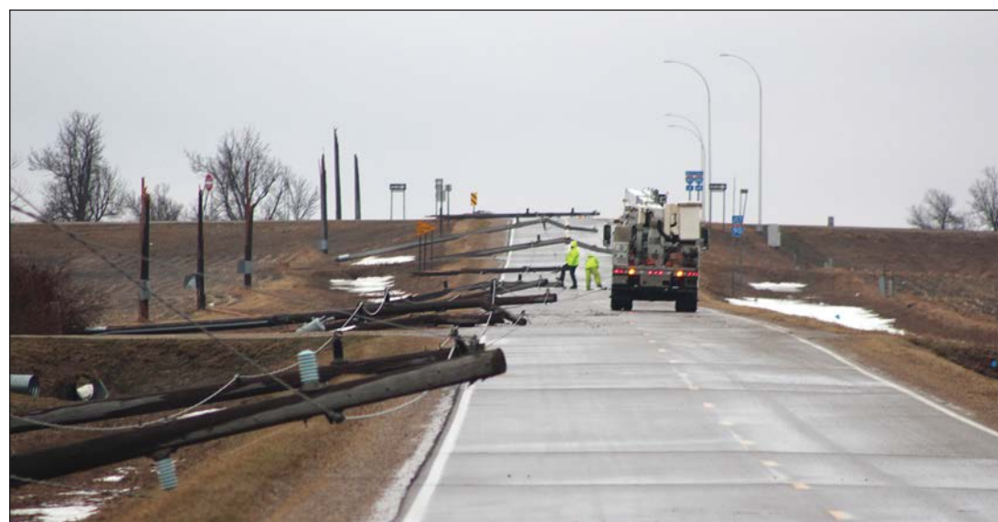
This photograph was taken around mid-day Friday of snapped power poles lying over County Road 3 near Magnolia to the south of the overpass facing north.
