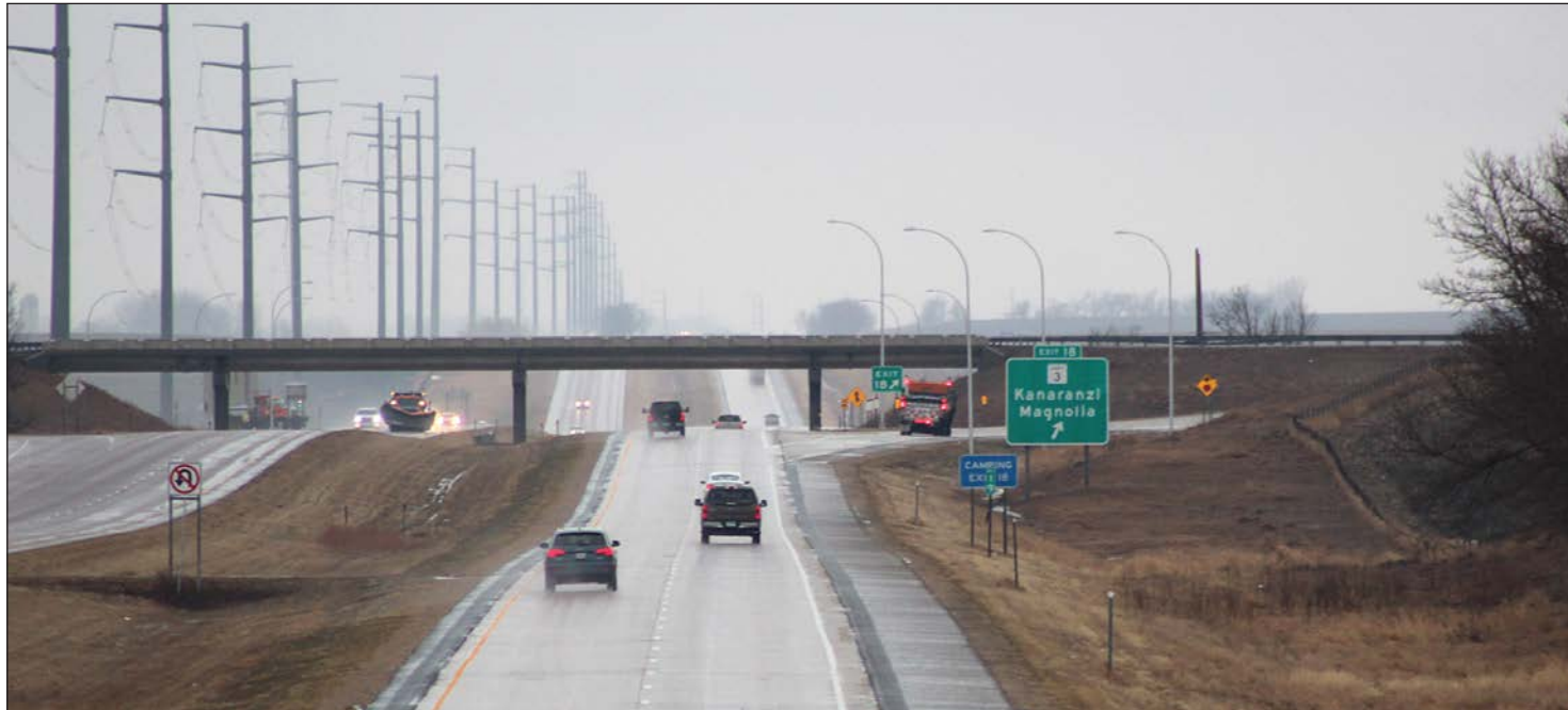
When snapped power poles lay across County Road 3 on the I-90 overpass, Magnolia exits were blocked from both directions until Monday. Sioux Valley Electric estimated $500,000 to replace the 60-70 power-line poles damaged by high winds.
