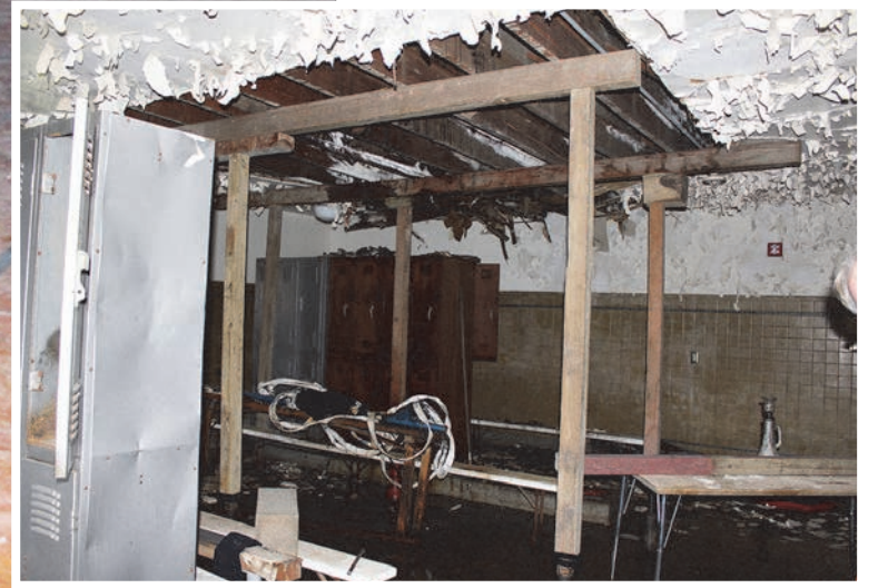
Below: The boys' locker room has suffered the most damage over the years from a roof leak. Workers have raised the ceiling within two inches of the roof.
