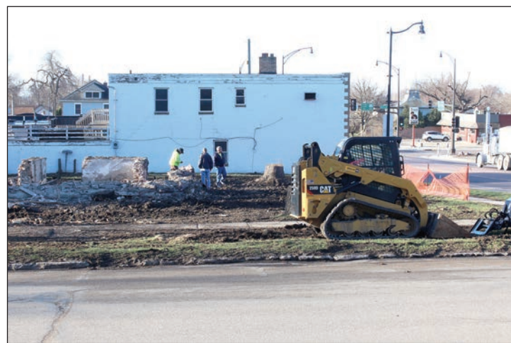
Lori Sorenson photos/0406 ramage house demolition
