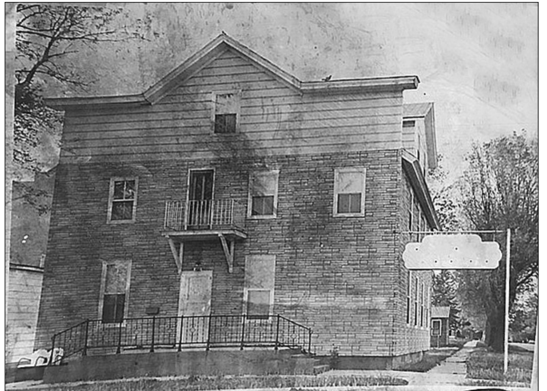
Current Senior Center building started out as Lincoln Hotel in 1880s in Luverne
