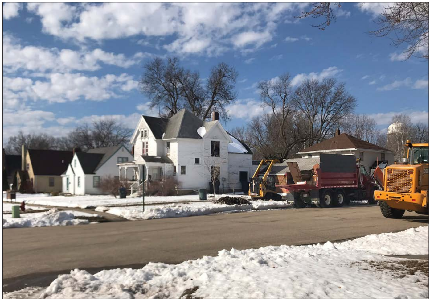
Lori Sorenson photos/0405 demolition at 319 north freeman
