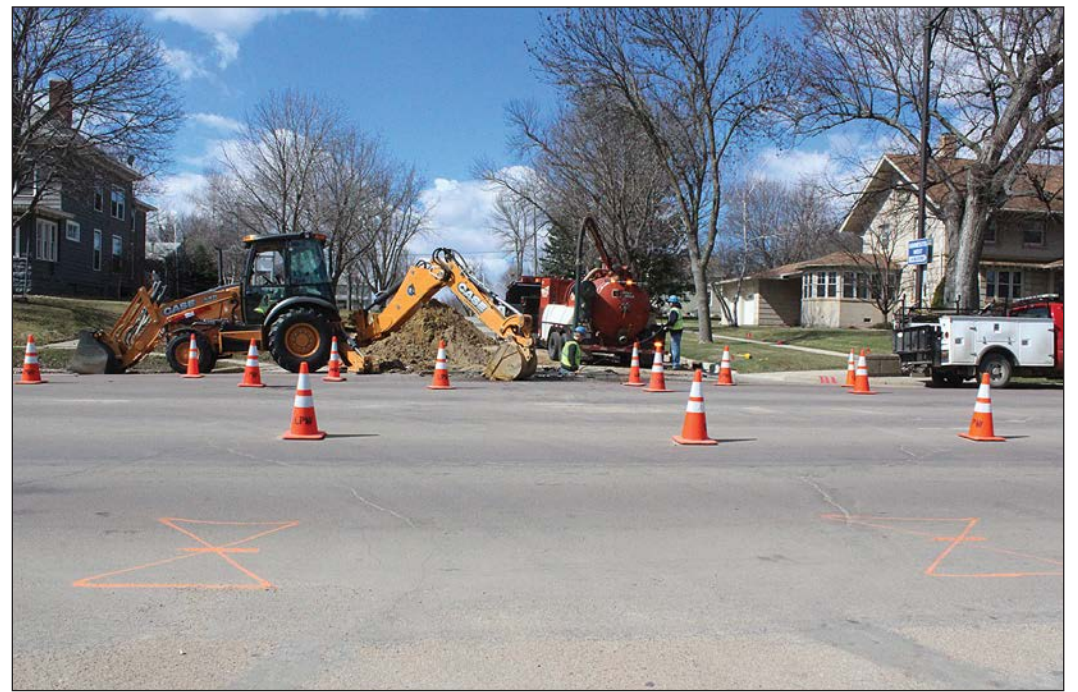
Lori Sorenson photo/0331 sewer repair
