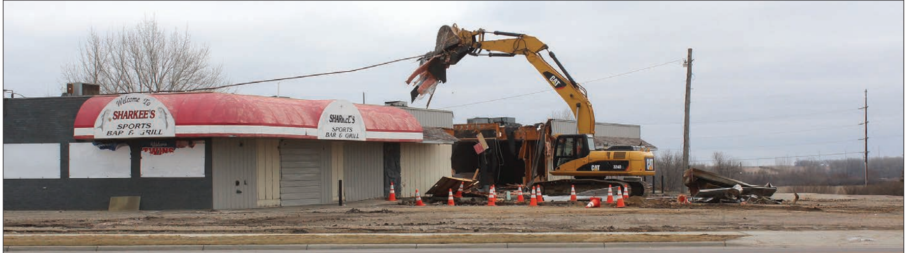
Lori Sorenson photo/0330 sharkee's demolition
