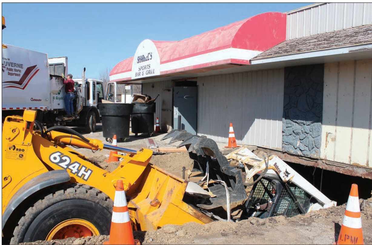
Lori Sorenson photo/0309 sharkee's demolition
