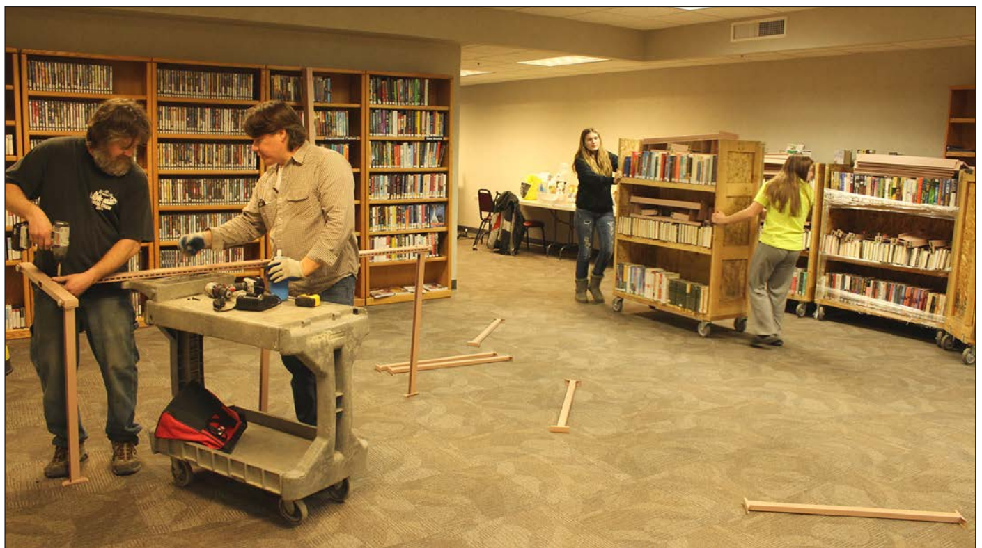
Mavis Fodness photo/0128 Library Renovation
