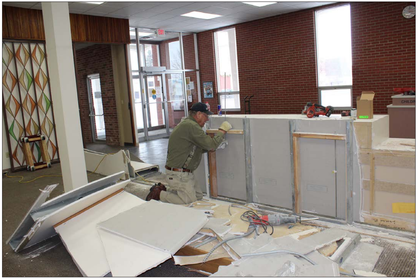
Mavis Fodness photo/0128 Library Renovation
