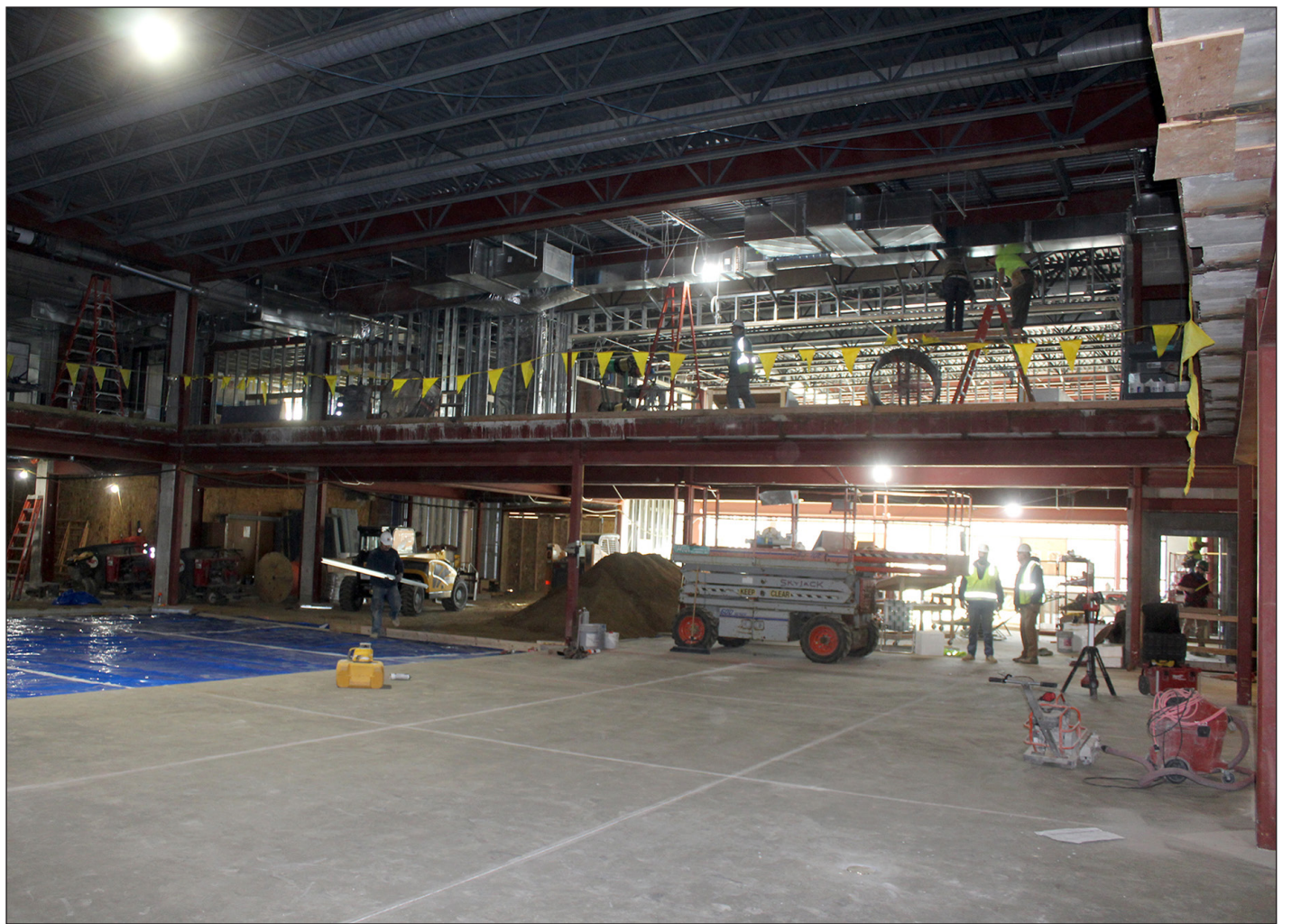
Mavis Fodness photo/1231 School Build Commons Facing South
