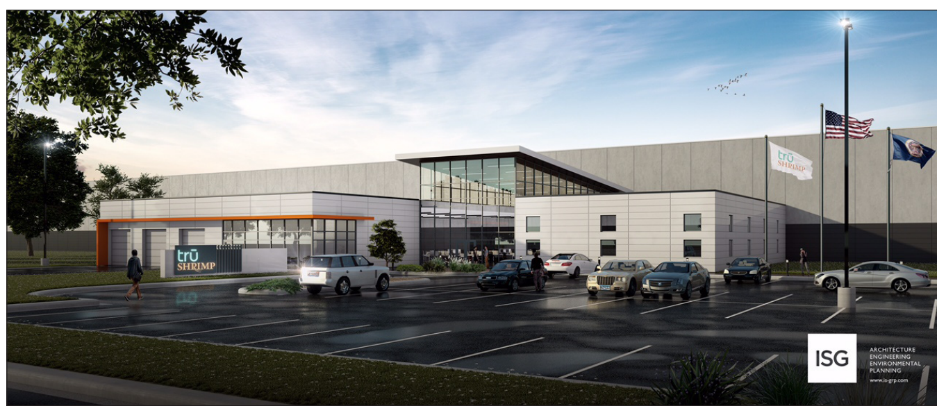
Tru Shrimp remains the shining star in the local economic development scene with more than $100 million in construction and 100 jobs on the horizon. The combination of the harbor, hatchery and accompanying water, electrical and gas distribution facilities are planned for 60 acres along the north side of I-90 in Luverne's industrial park.
