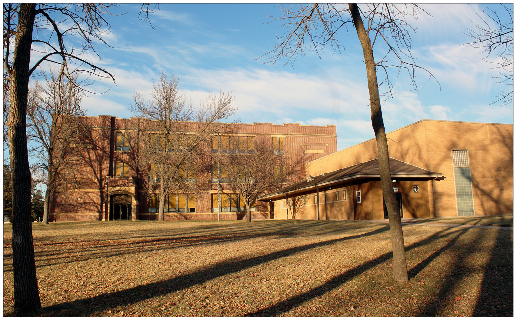
Mavis Fodness photo/1210 HBC Facilities Assessment
