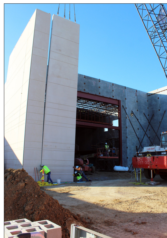
A 56-foot precast concrete panel is lifted into place Monday for the back wall of the performing arts center at the school. The addition is expected to be fully enclosed this month.
