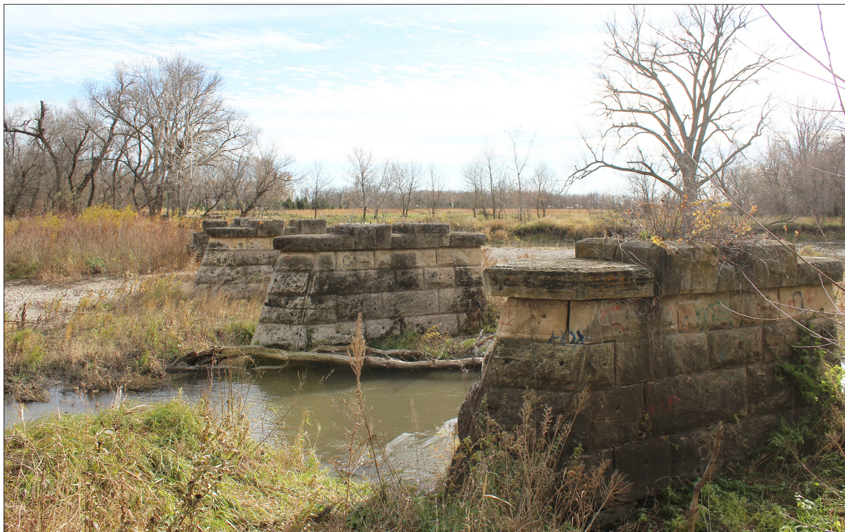
Mavis Fodness photo/1118 Rock River Bank Project
