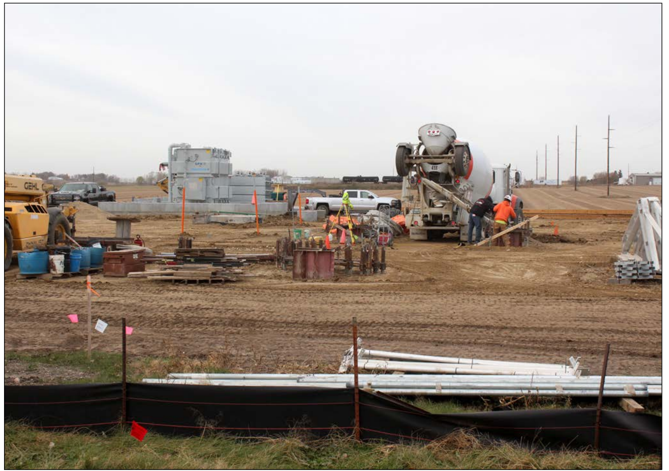
Lori Sorenson photo/1101 transformer work
