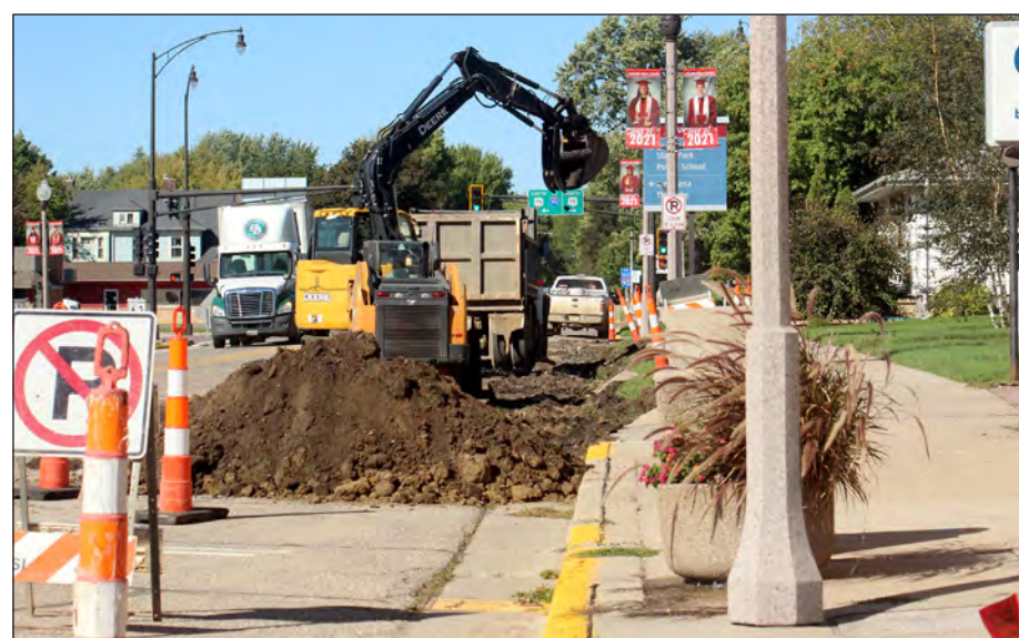
Crews with Musch Construction, Pipestone, work on Main Street Friday.
