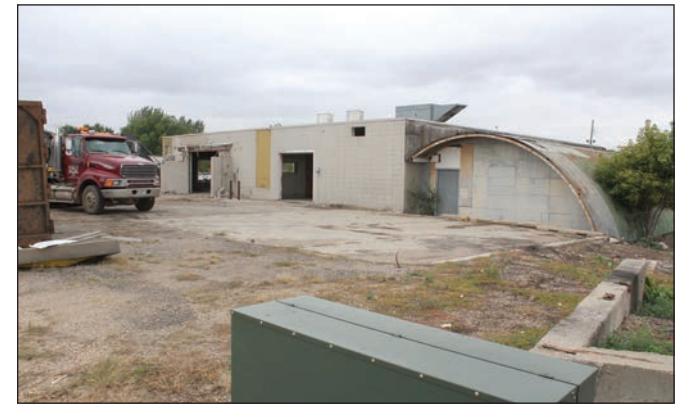
Lori Sorenson photo/0927 china inn demolition
