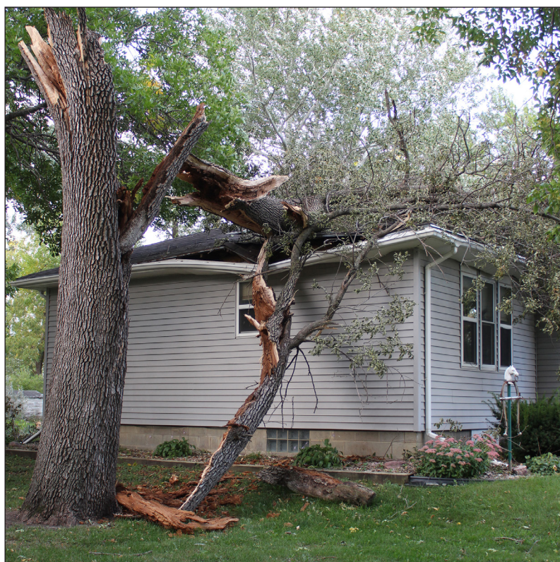
Mavis Fodness photo/0923 Storm Damage 9-17
