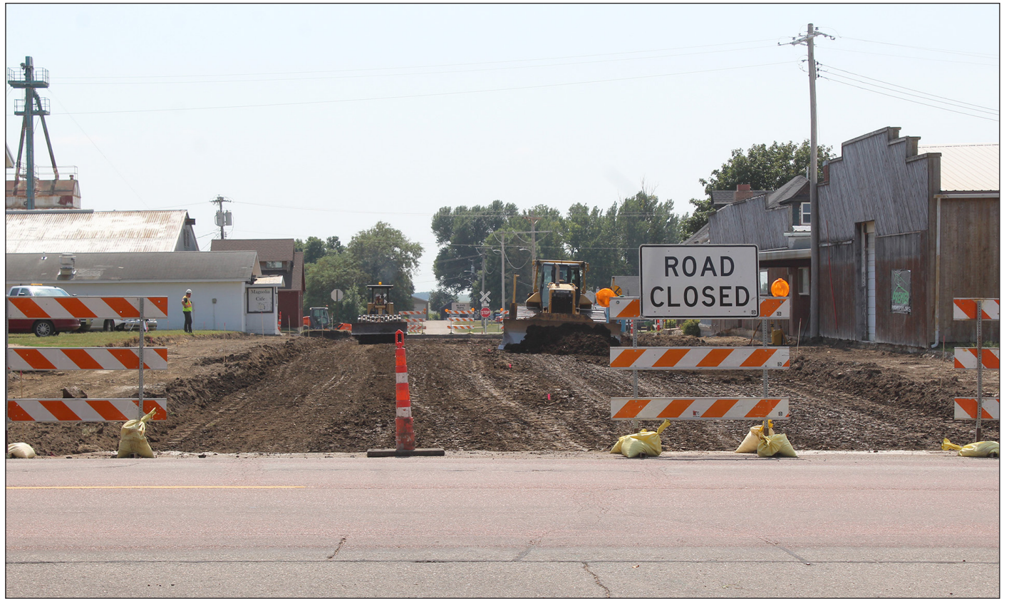
Mavis Fodness photo/0903 Road Construction Magnolia
