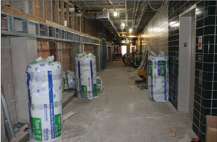
Mavis Fodness photos/0829 School Build West Wing Before
