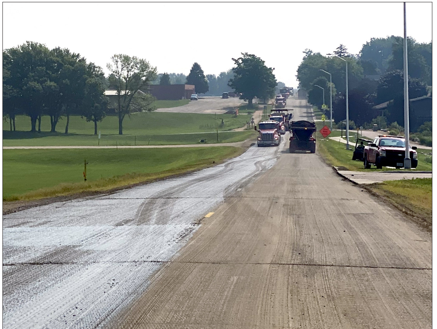
Lori Sorenson photo/0804 Dodge Street work
