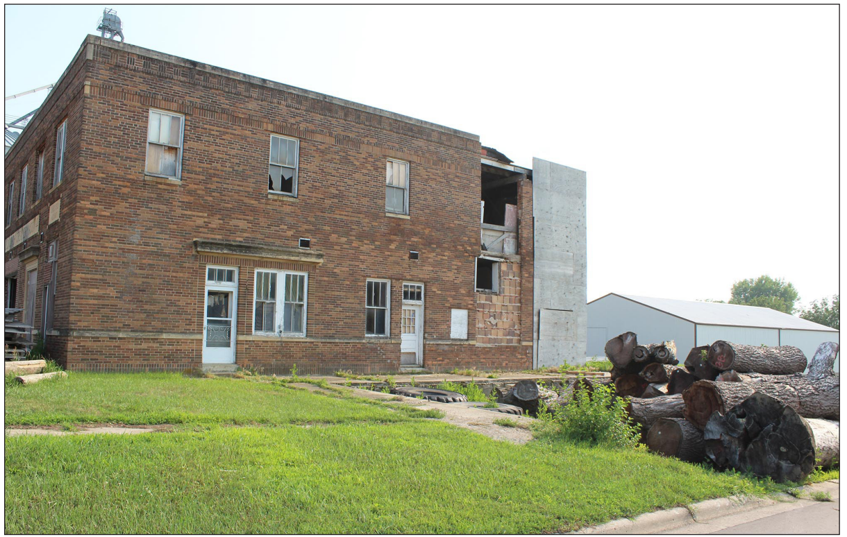
Mavis Fodness photo/0722 Hills Creamery Demolition
