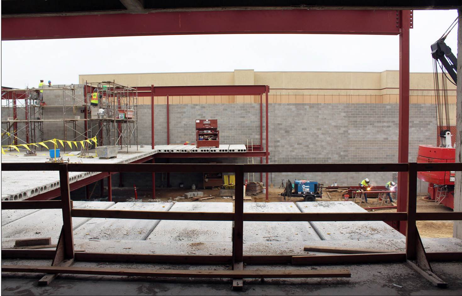
Mavis Fodness photo/0709 School Build July 2020
