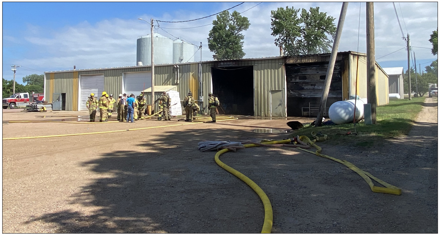
A July 4 fire caused extensive damage to the Hills Storage Center and destroyed a semitrailer owned by Harlan and Sue Stueven, Hills. No one was injured, and the cause of the blaze is being investigated. (Lori Sorenson photos)
