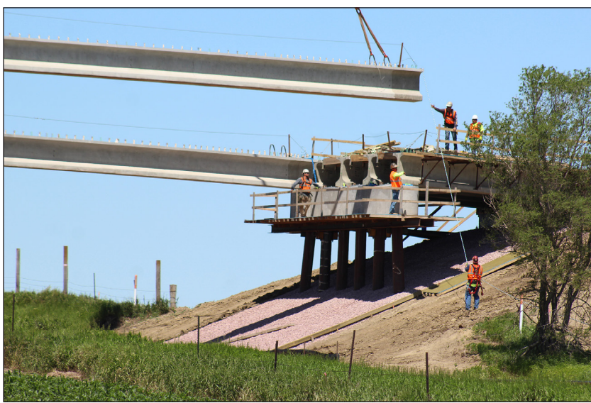
Above, workers guide a large concrete beam that the crane places over the BNSF railroad. At right, Prahm Construction workers attach the 106-foot-long concrete beam into place as the operator from Barnhart crane division waits to lift the second of four beams into place.
