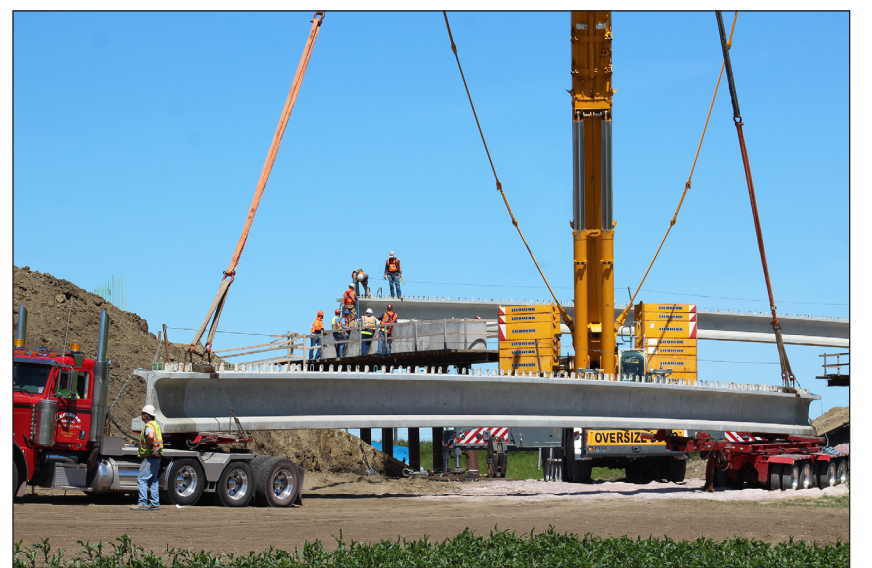
Above, workers guide a large concrete beam that the crane places over the BNSF railroad. At right, Prahm Construction workers attach the 106-foot-long concrete beam into place as the operator from Barnhart crane division waits to lift the second of four beams into place.
