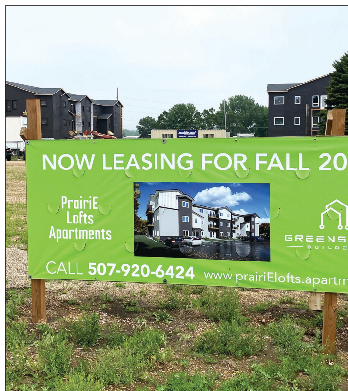
The current black exterior is a sprayed on barrier, used instead of Tyvek. It's "waterproof, weather- and vapor-resistant, UV stable and eco-friendly," according to GreenSmith Builders.
