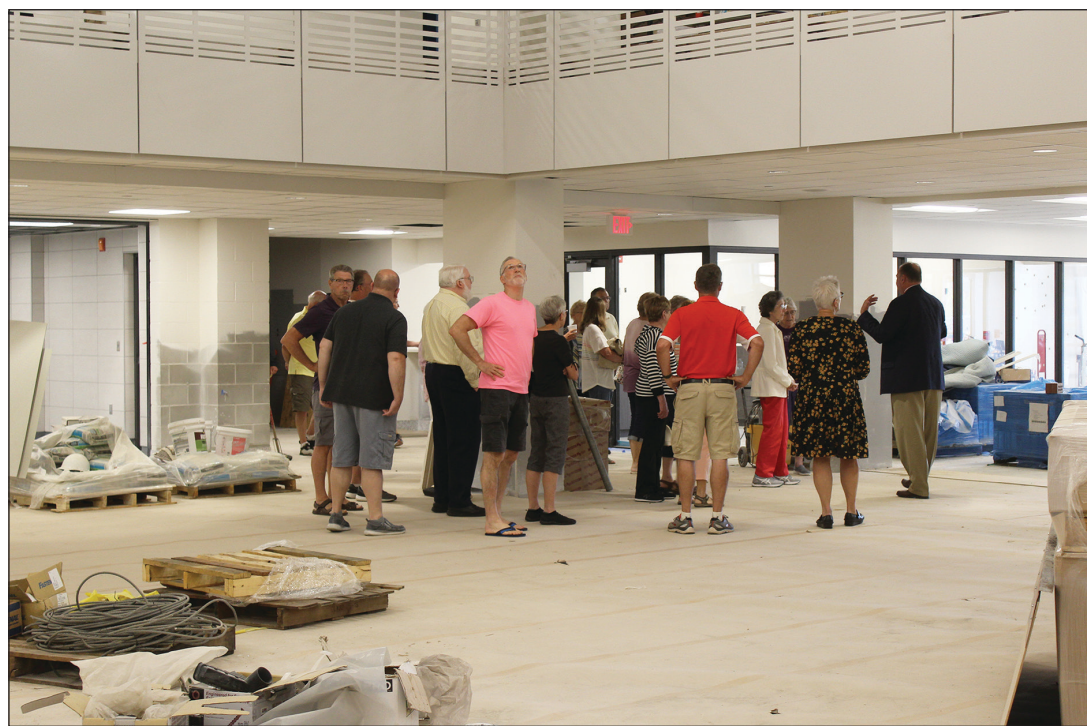
The new commons at the Luverne Middle-High School can accommodate 411 students.
