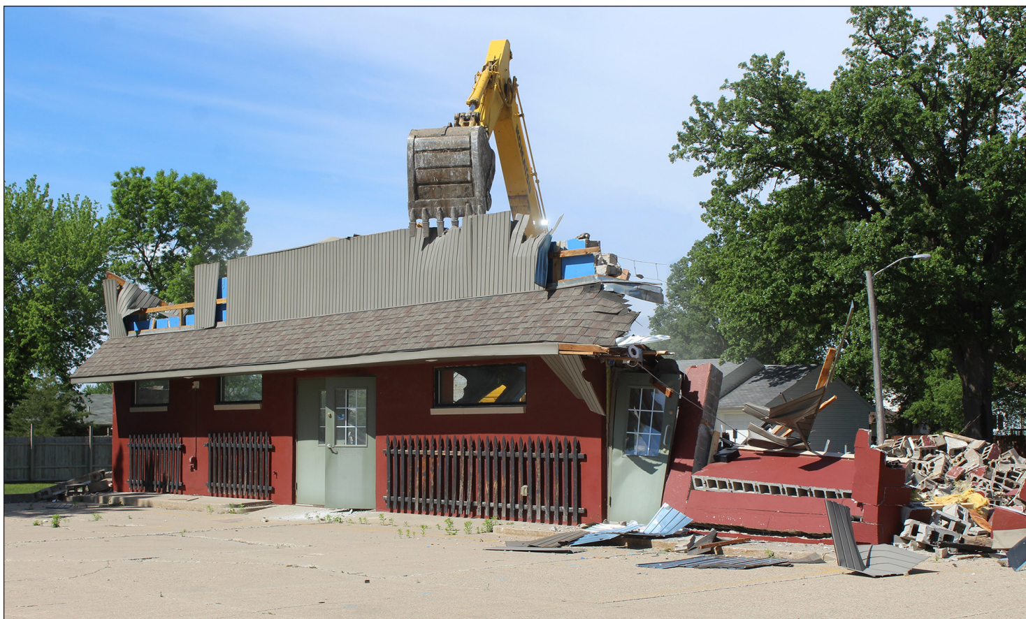
Mavis Fodness photos/0609 remede demolition
