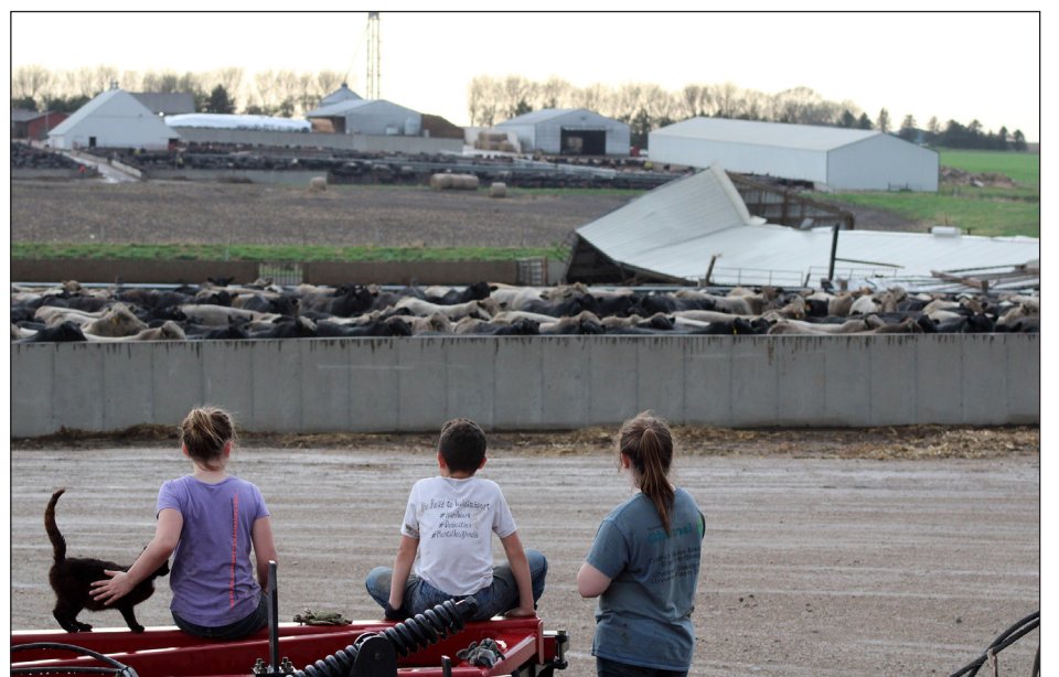
Lori Sorenson photos/0519 storm damage
