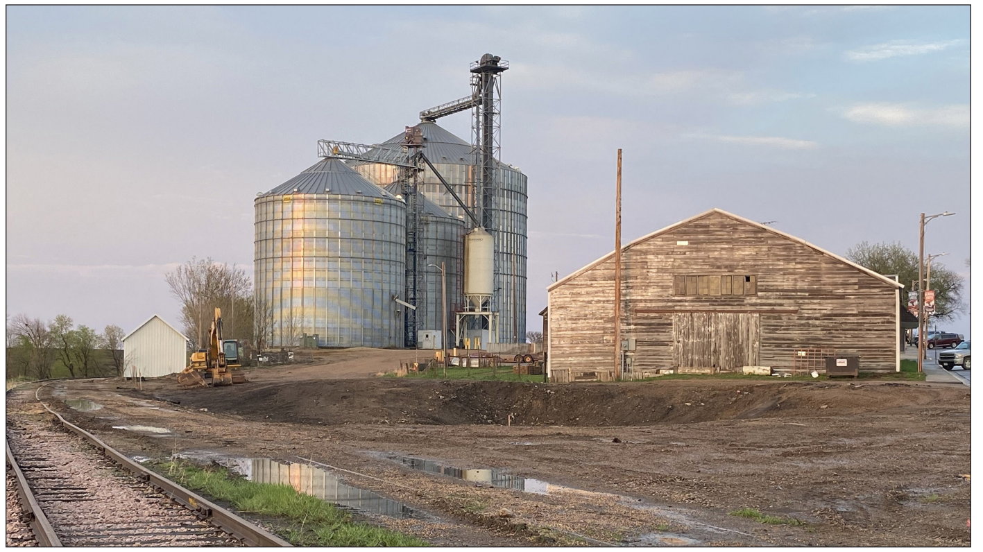
Lori Sorenson photo/0519 beaver creek elevator lot
