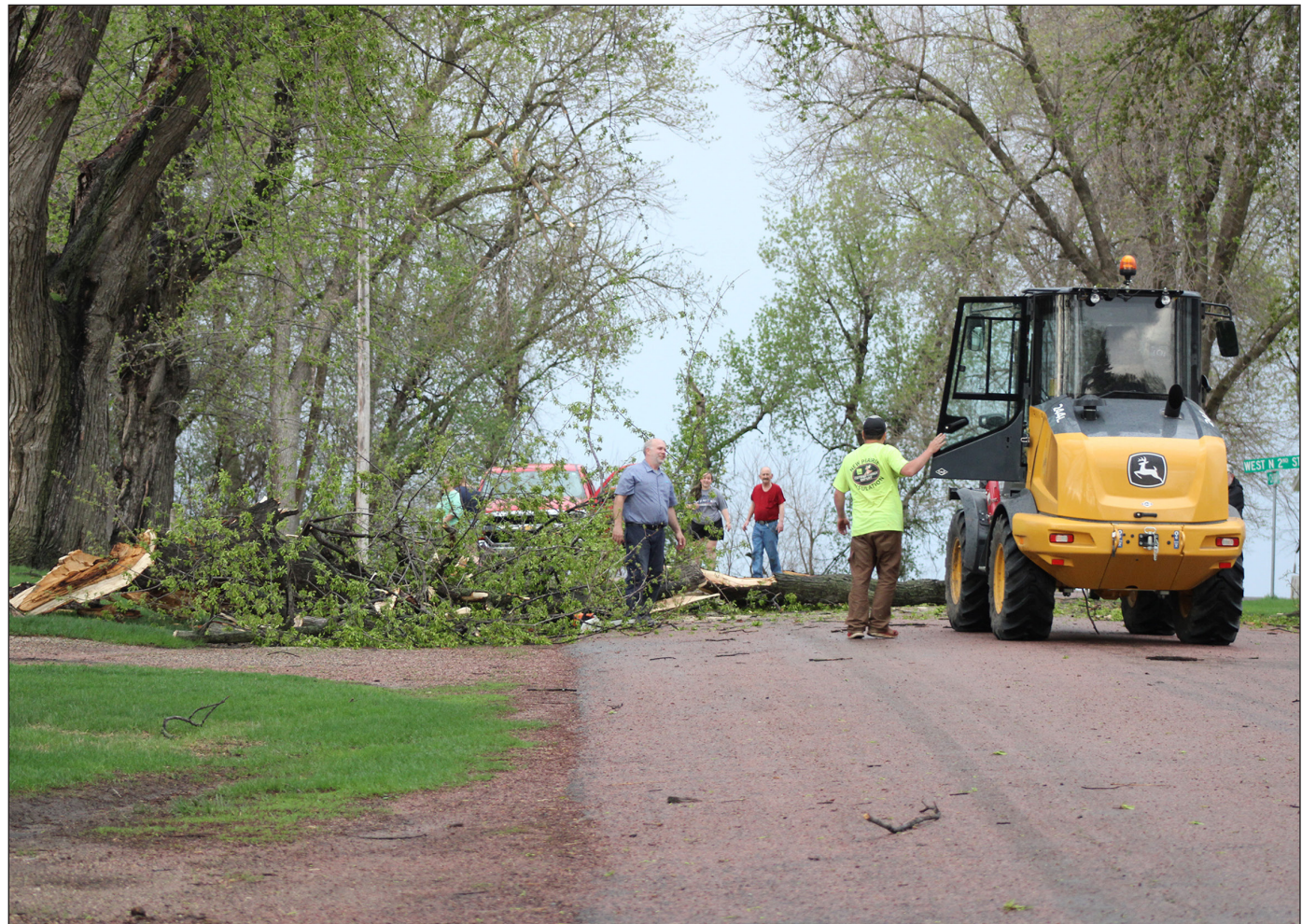
Lori Sorenson photos/0519 storm damage
