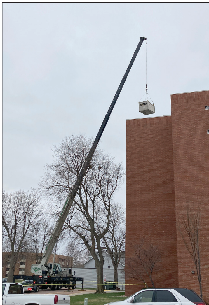
Esther Frakes photo/blue mound tower crane
