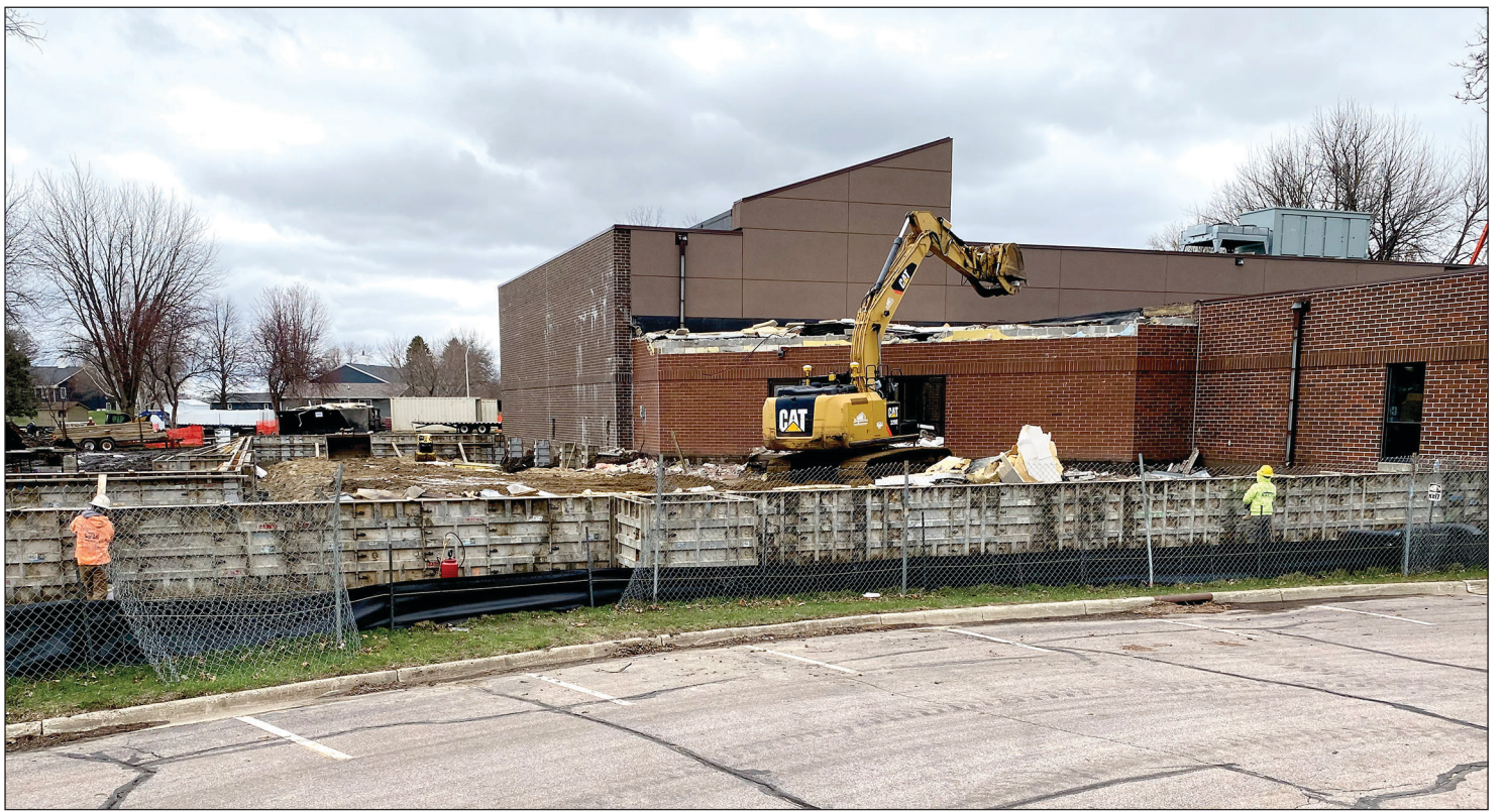
Lori Sorenson photos/0422 pool and fitness construction
