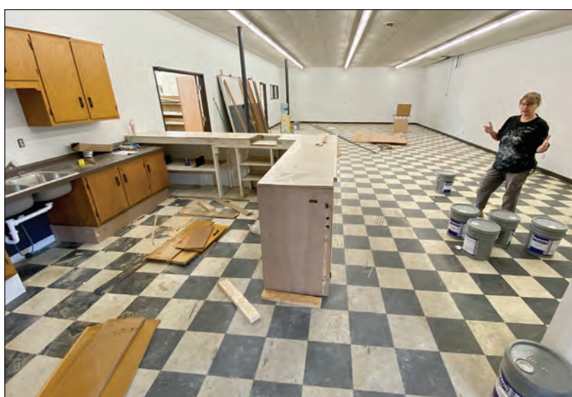
Lori Sorenson photo/0225 ATLAS construction
