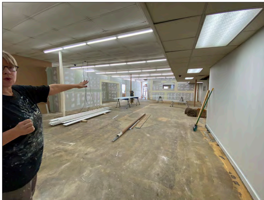
Lori Sorenson photo/0225 ATLAS construction
