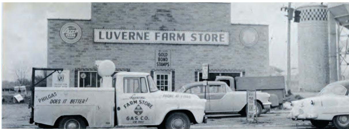
ATTRACTIVE is this exterior of Luverne (Minn.) Farm Store. The warehouse is shown to the rear.
