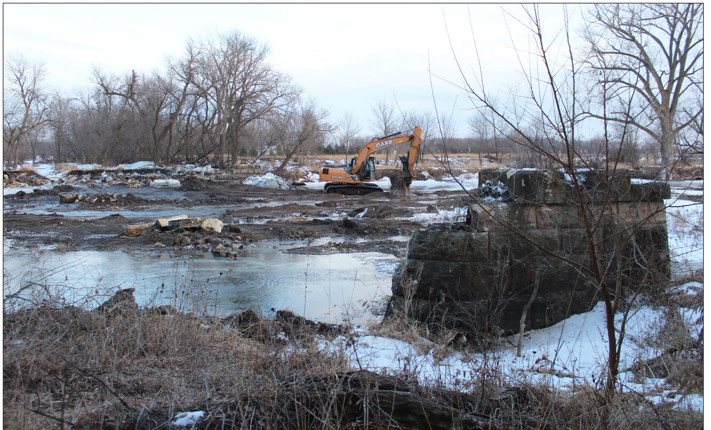
Mavis Fodness photo/0204 Pillar Removal
