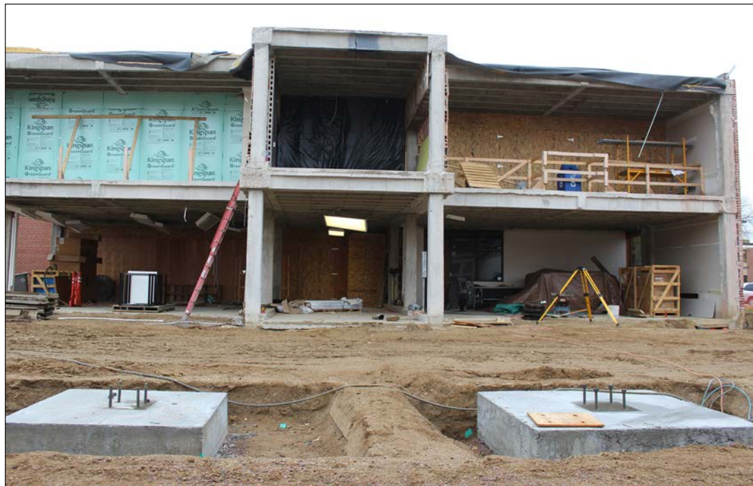
Mavis Fodness photo/1024 School Build West Wing End
