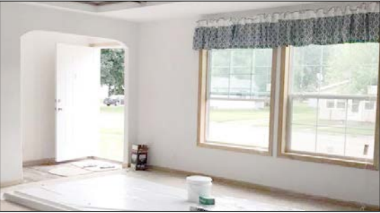
Above, workers finish siding Ykema’s manufactured home after the two sections were placed on a new foundation and joined together. At left are Jill, Darrel and Michael (in front). Below, the home features arched doorways.
