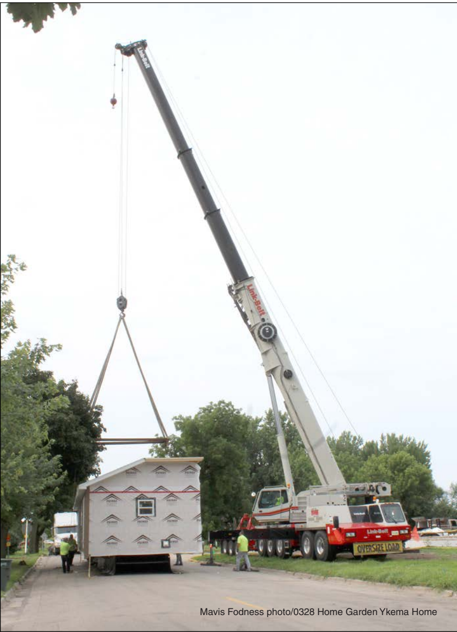
Pictured at left a crane lifts one half of Darrel and Jill Ykema’s manufactured home into place on its new foundation on South Donaldson Street in Luverne July 2018. The Ykemas chose the home for its quick design and construction processes.
