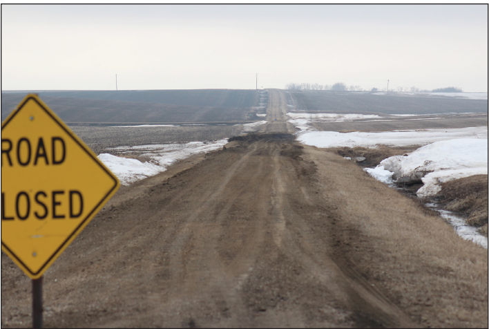
Mavis Fodness photo/0328 Gravel Roads 2019 Battle Plain Some township gravel roads such as this one in Battle Plain Township remain closed due to the spring snowmelt leaving the road surface soft. of township roads as possible." It's the first time in the store's 71-year history that deliveries from its feed mill began at 4 a.m. instead of the traditional 8 a.m. Golla estimates at least
