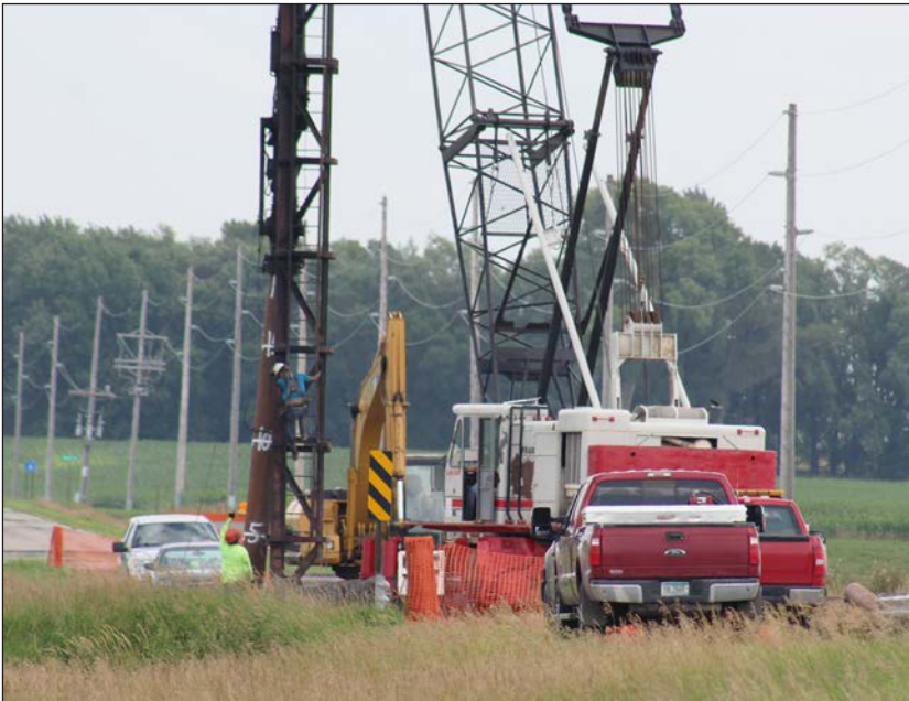
Steel replaces wood pilings that were damaged by ice flow this spring. Transfer girders will also be replaced on the project that started July 15.
