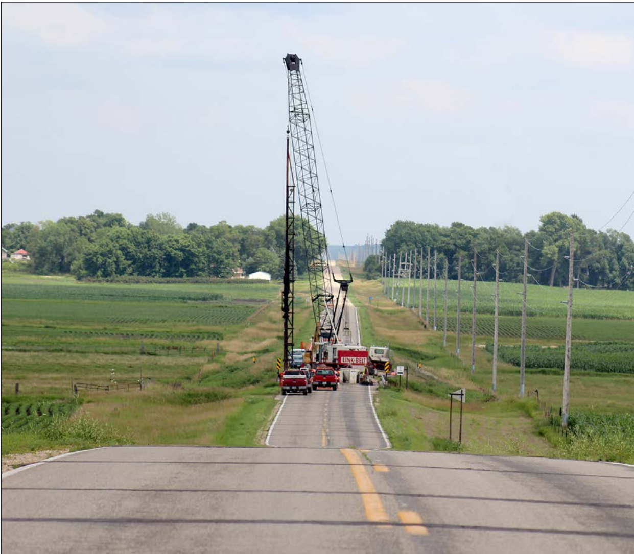
Workers from Prahm Construction, Slayton, use a crane to install steel pilings for the County Road 1 bridge over Kanaranzi Creek in southeastern Rock County. Work is expected to be finished by the end of the week.
