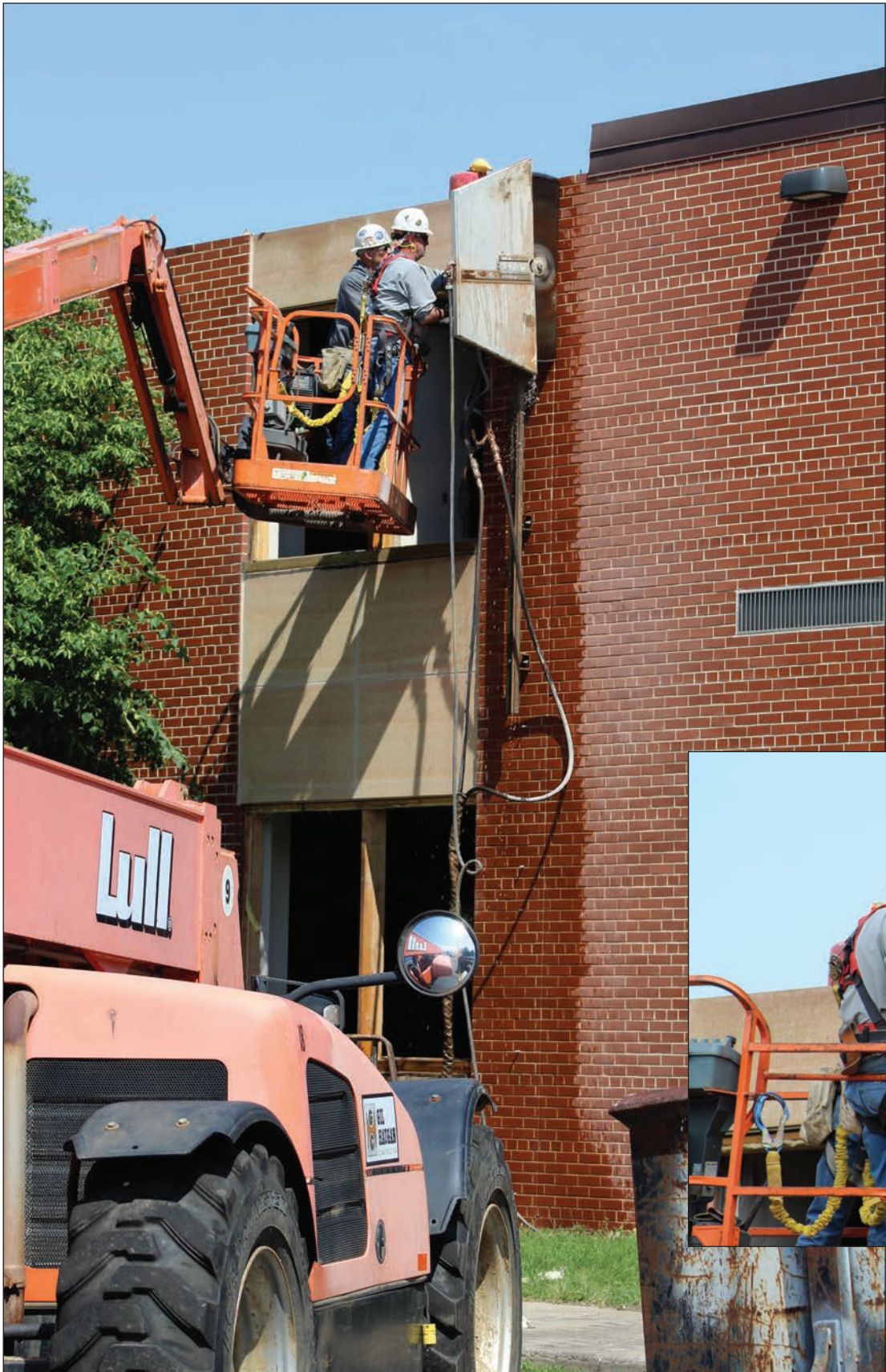
Mavis Fodness photo/0620 School Project June 2019 Joel Farrell (left) and Jim Houten with Gil Haugan Construction of Sioux Falls position the 48-inch saw blade into position Thursday morning, June 13, at the Luverne Middle-School High School.
