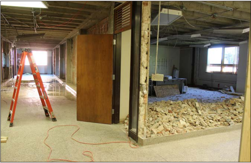
Classroom walls are removed in the first floor of the west wing in Mark Lundgren's former classroom on the north side of the hallway.
