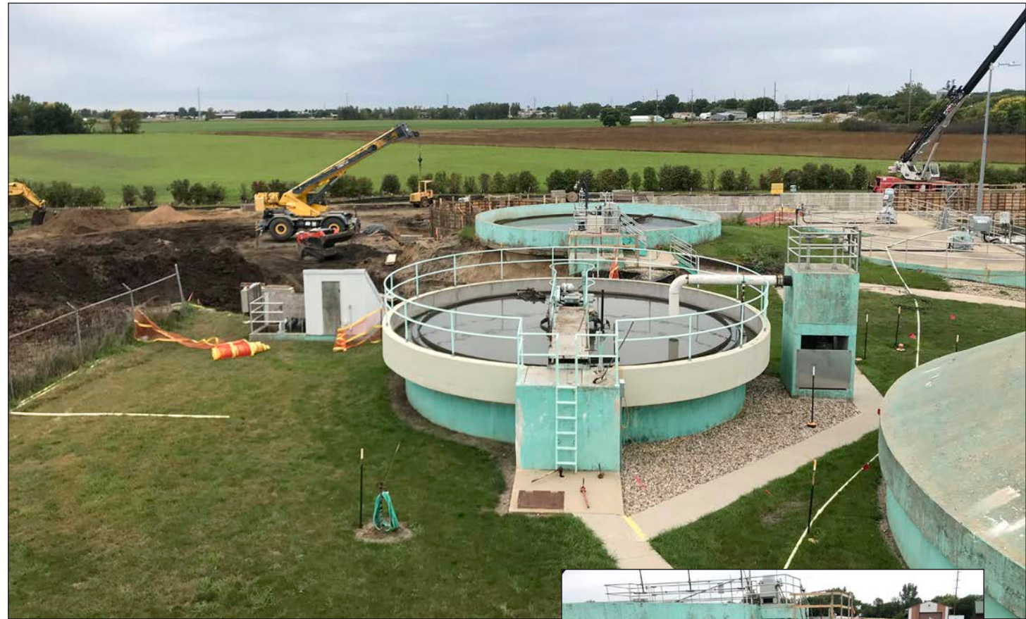
A new primary clarifier will join an existing one on the west and south end of the campus, and a 1960s clarifier to the east will be removed. At right, footings are poured for the new splitter box, which takes in wastewater flow and splits it to each of the clarifiers to moderate workload both ways.
