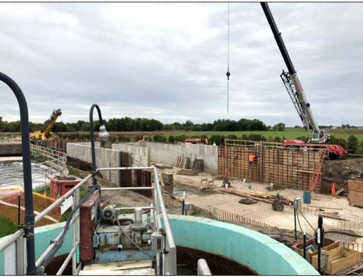
Lori Sorenson photos/1003 wastewater treatment plant construction6 The foundation and walls of the new oxidation ditch are poured next to the existing oxidation ditch. This photograph is taken from the north end. Solid waste flows continuously through the unit, which uses forced air and bacteria to break down solids.
