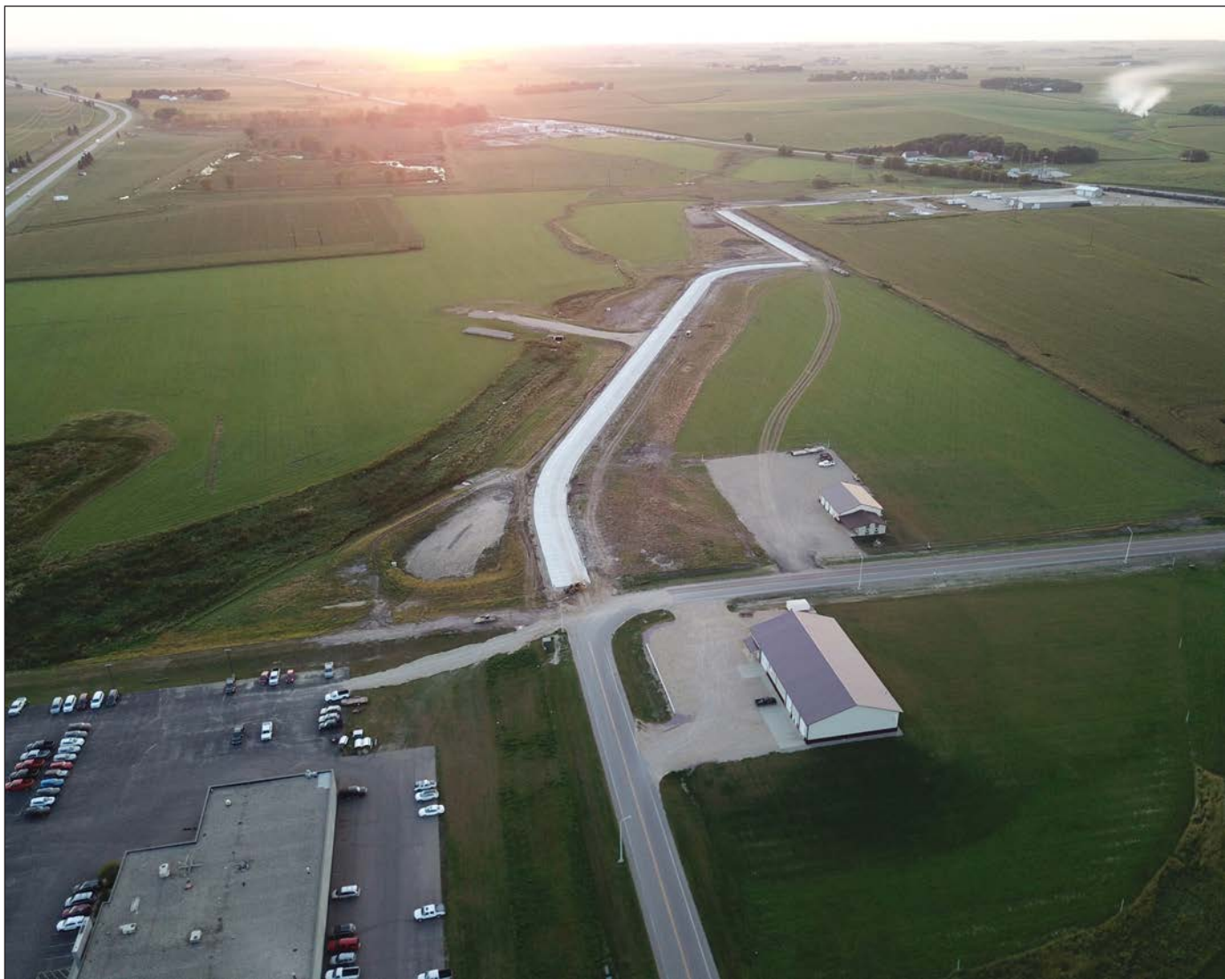
Luverne drone enthusiast Ryan Gee shared this image of Luverne's industrial park several weeks ago as Koehn Avenue was being paved to meet Minnesota Avenue to the west. It is a 10-ton road to accommodate industrial growth.
