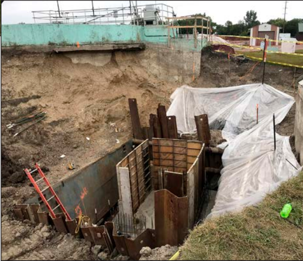
A new primary clarifier will join an existing one on the west and south end of the campus, and a 1960s clarifier to the east will be removed. At right, footings are poured for the new splitter box, which takes in wastewater flow and splits it to each of the clarifiers to moderate workload both ways.
