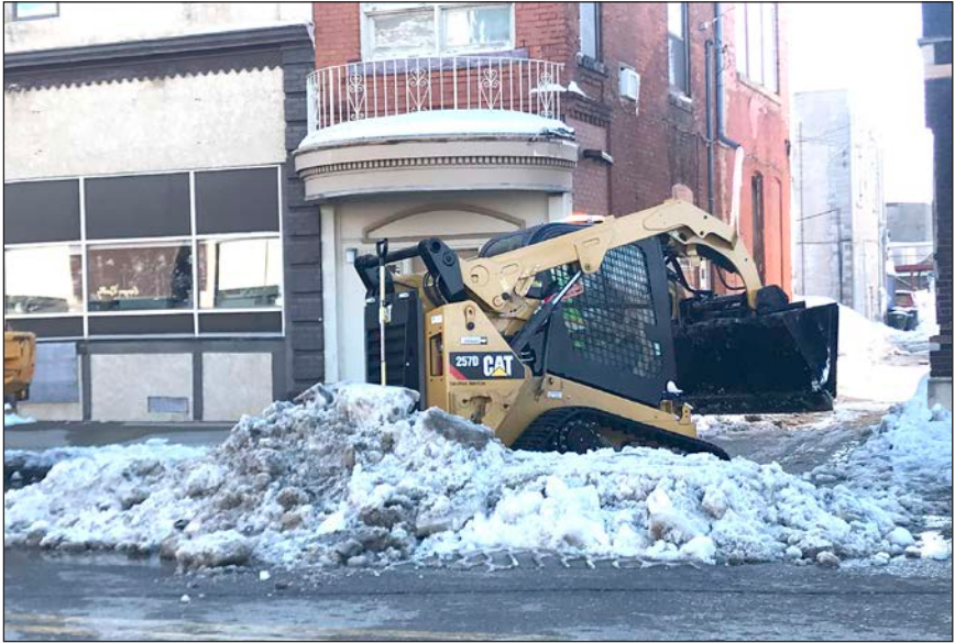
Lori Sorenson photo/0314 clearing storm gutters City crews pull snow and slush from the alley off Cedar Street Monday. They put in extra hours to clear storm gutters and streets to make room for heavy rain — and possible flooding — forecast for later this week.
