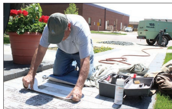
Vance Walgrave carefully tapes the rubber stencil to protect the other pavers from the sandblasting.
