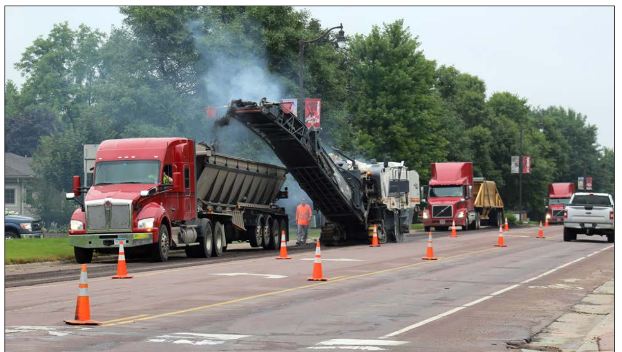
Mavis Fodness photo/0815 highway 75 repairs
