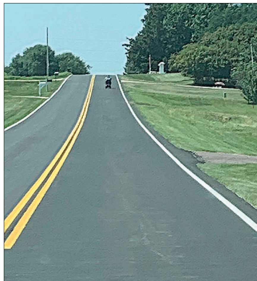
With pedestrian walkways prevalent around the city of Luverne, West Warren Street falls short and as a result pedestrian visitors are forced to use the roadway to get to Maplewood Cemetery.
