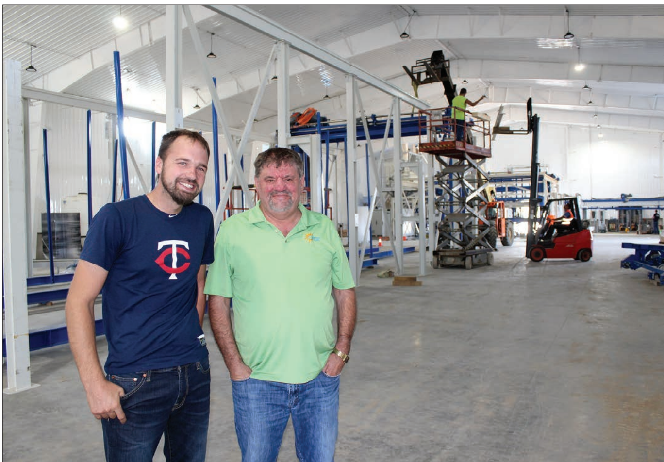
Mavis Fodness photo/Ag Tab Midwest Dry Cast Aaron (left) and Melvin Waldner, pictured in the east end of the Midwest Dry Cast building currently under construction south of Luverne, operate the SD Industries in Alexandria, South Dakota, and are working with a French company to assemble the equipment to produce agricultural concrete products. Plans are to produce floor slats in Luverne for swine facilities beginning next month.
