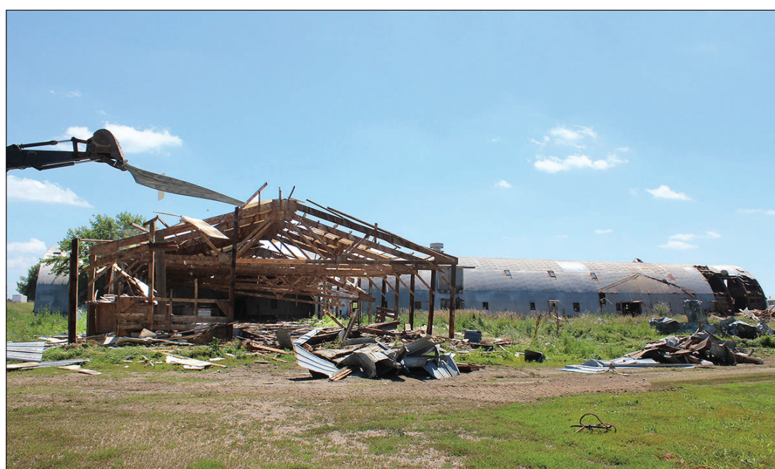
Stephanie Christensen photos/0730 turkey barns demolition
