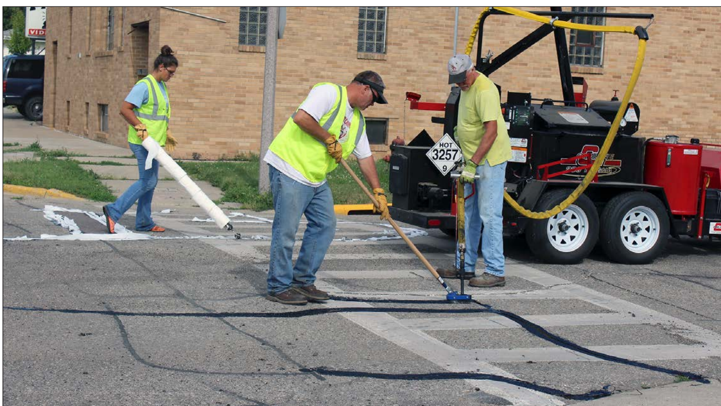
Mavis Fodness Photo/0721 City Street Repairs
