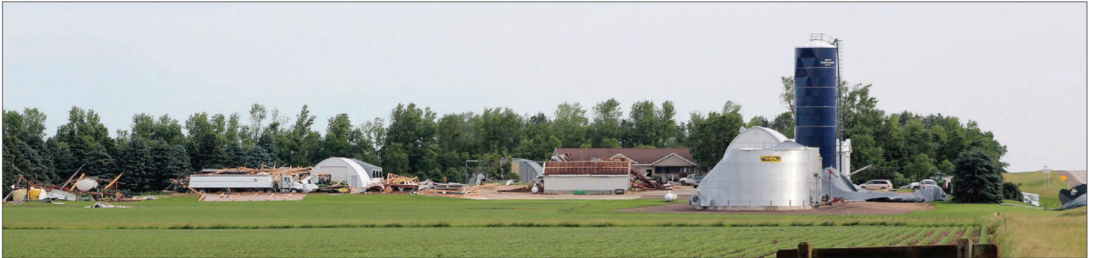
Lori Sorenson photo/0625 storm damage veldkamps
