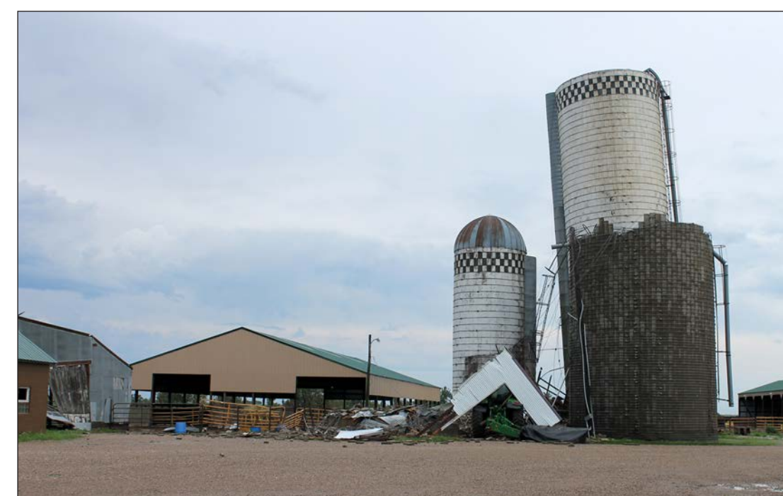
A portion of an estimated 60-foot-tall stove silo toppled and another silo leans to the southeast at the J.R. Scott farm east of Hardwick where employee Cory Madson lives. No people or livestock were injured. The damage was caused by a half hour of northwest winds in excess of 50 mph that went through the area early Monday morning. (Mavis Fodness photo/0625 storm2)
