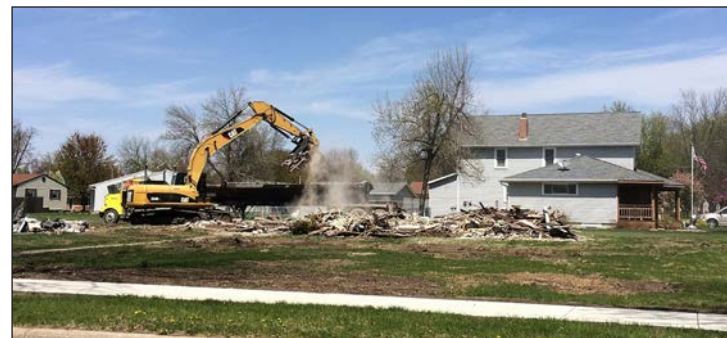
Chantel Connell photo/0507 barck demolition
