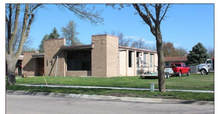
Lori Sorenson photo/0507 barck demolition
