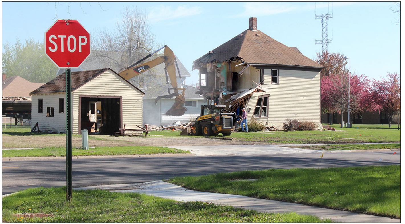
Lori Sorenson photo/0507 barck demolition
